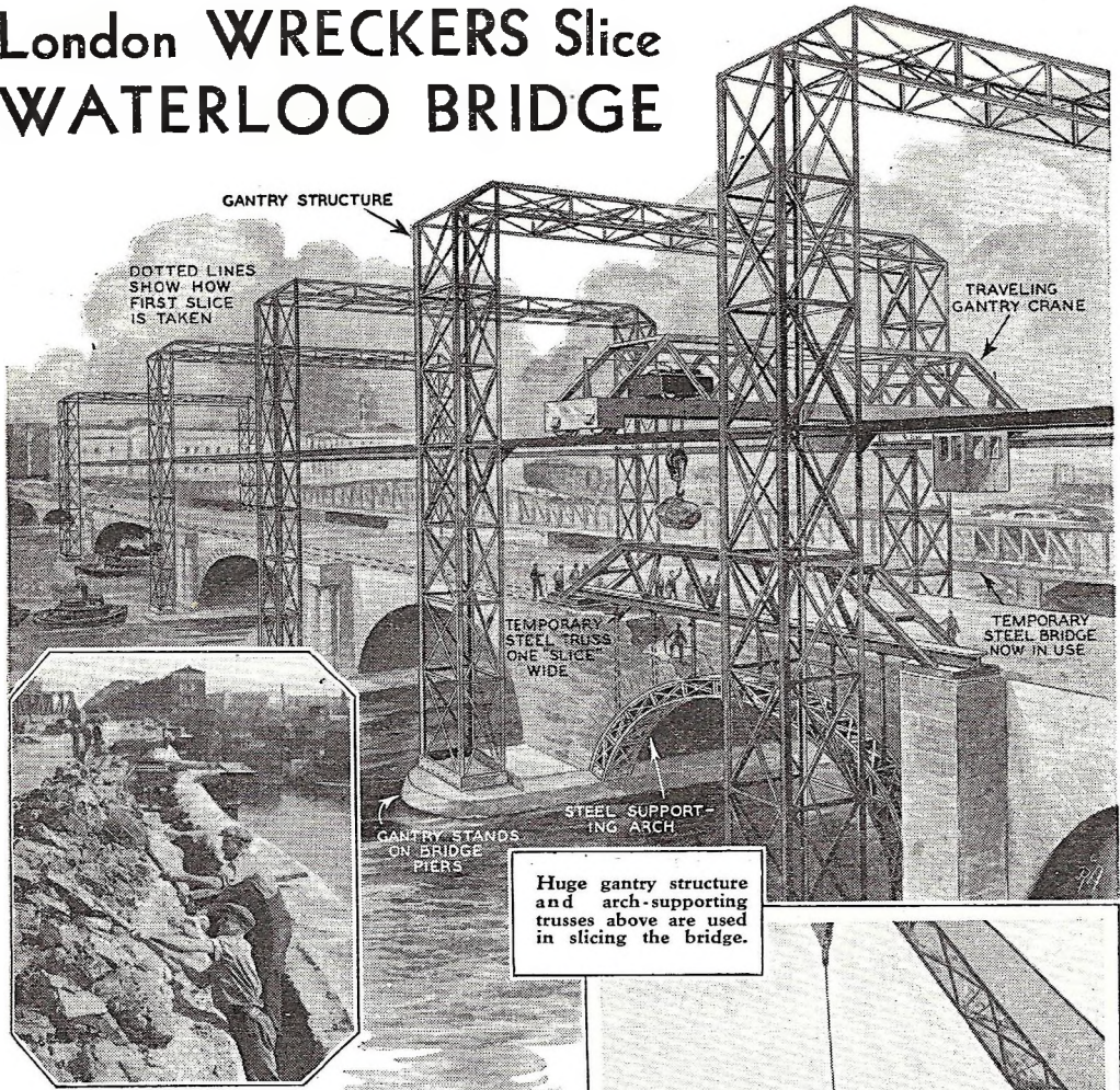
Beds of clay just above arches of Waterloo bridge have, after 123 years, become hard as iron and difficult to remove.
